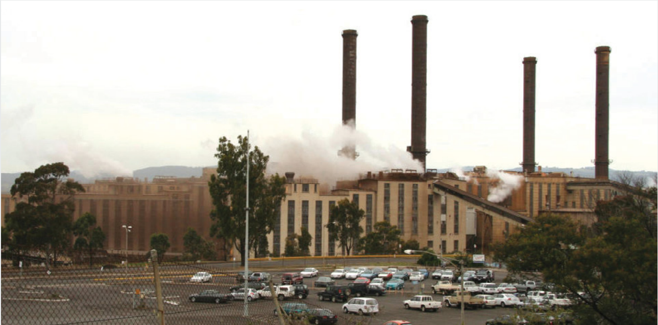
EnergyBrix / Morwell Power Station. Source: Wikipedia
