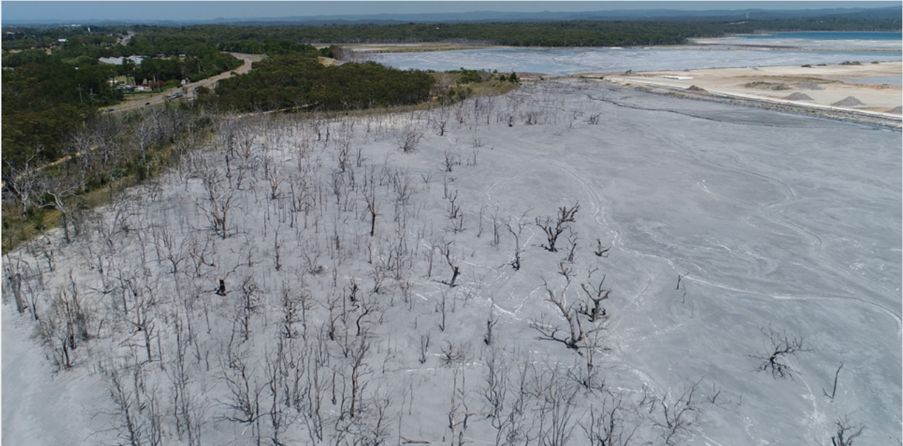
Vales Point ash dump from above, NSW Central Coast. Source: supplied
