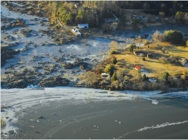
Coal ash dump collapse, Tennessee, US, 2018. Source: Dot Griffith photography
