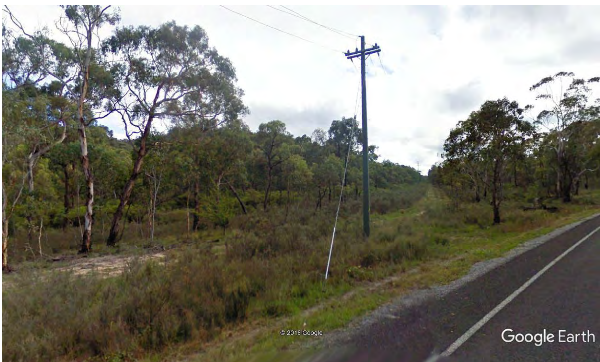
Figure 2.16: Utilities corridor parallel to Wolgan Road – looking northeast (StreetView image from Google Earth, 2018)
