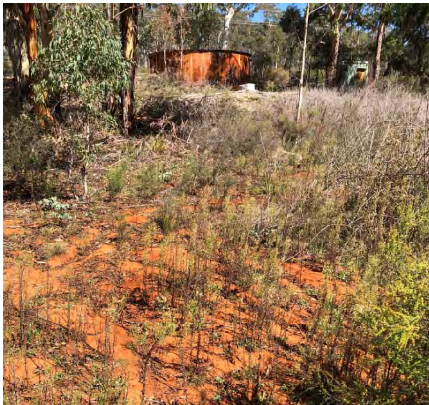
Figure 4-2 Invincible dewatering infrastructure
